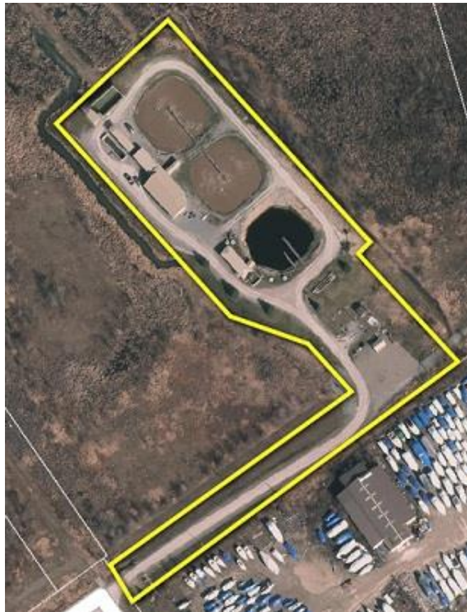
(Infrastructure – Item j – 155 Laguna Parkway)
