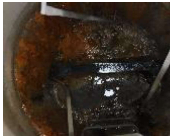
Figure 7: Infiltration in MH26 (left) and MH28 (right)
