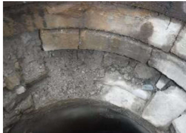
Figure 6: Grade Adjustment in MH47
