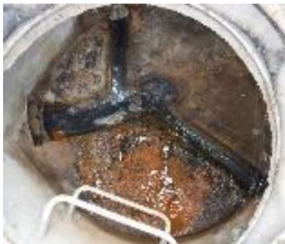
Figure 7: Infiltration in MH26 (left) and MH28 (right)
