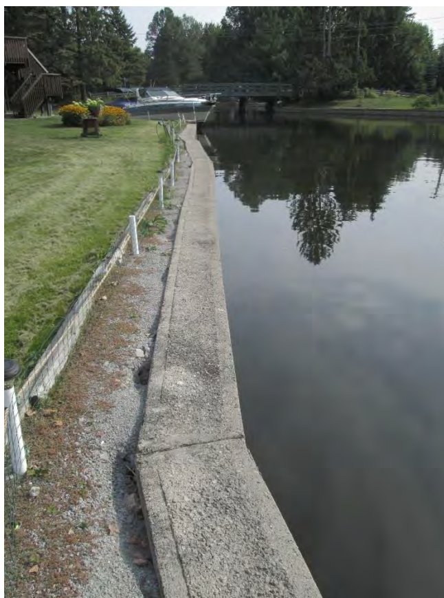
Photograph No. 6 Minor erosion (isolated spillways) behind wall.
