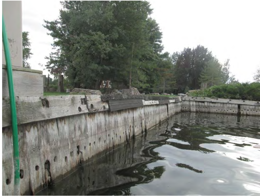
Photograph No. 3 Leaning/bowing/splitting of wood planks.
