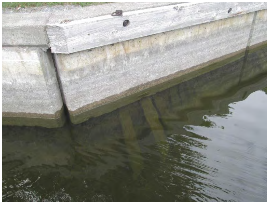
Photograph No. 2 Typical concrete fascia wall with wood planks behind.
