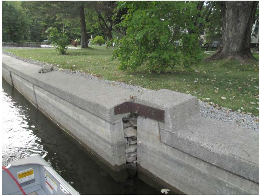
Photograph No. 15 Lateral movement in wall and repair detail.
