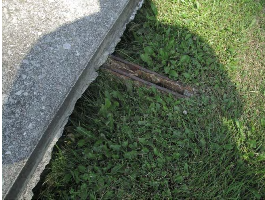
Photograph No. 21 Exposed tieback at grade with minor (surface) corrosion.
