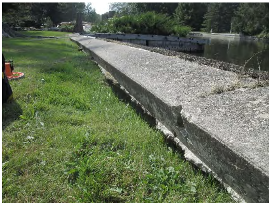
Photograph No. 5 Erosion and sloping of grade towards wall. Top cap tipping away from canal.
