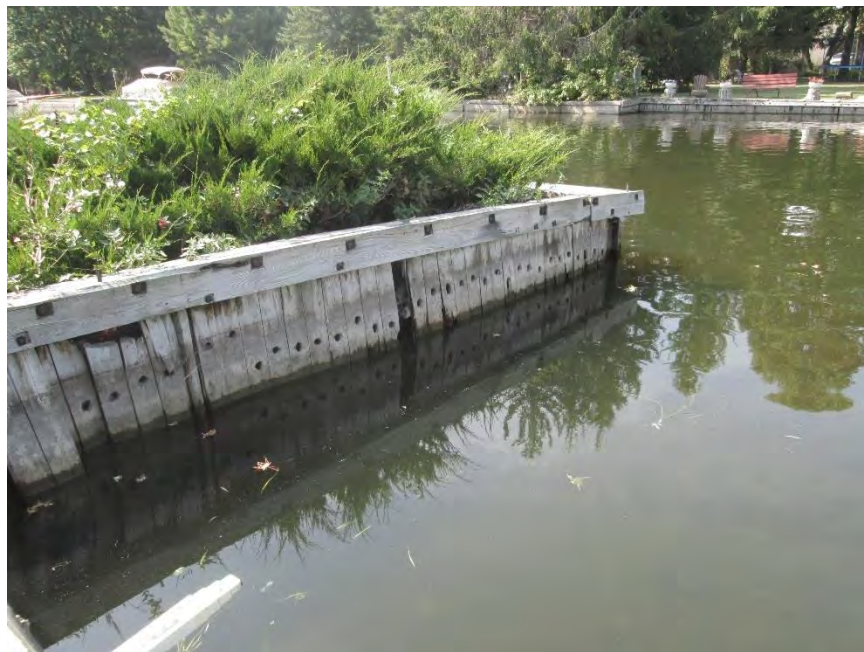
Photograph No. 4 Missing planks and exposed granular fill.
