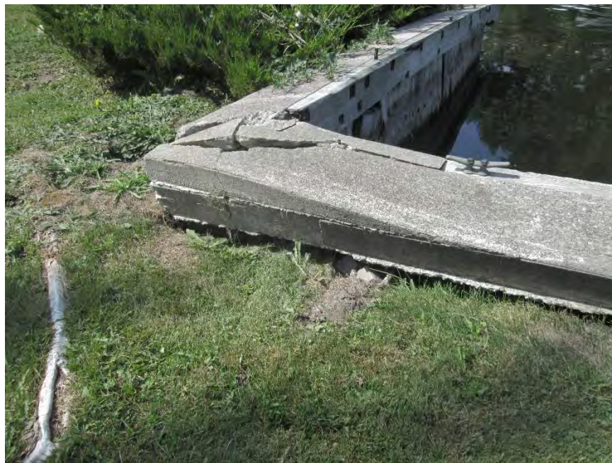
Photograph No. 12 Damaged top cap and erosion behind wall.
