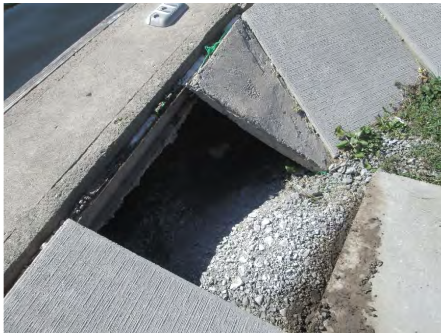
Photograph No. 8 Severe erosion behind wall – settlement of patio stones.
