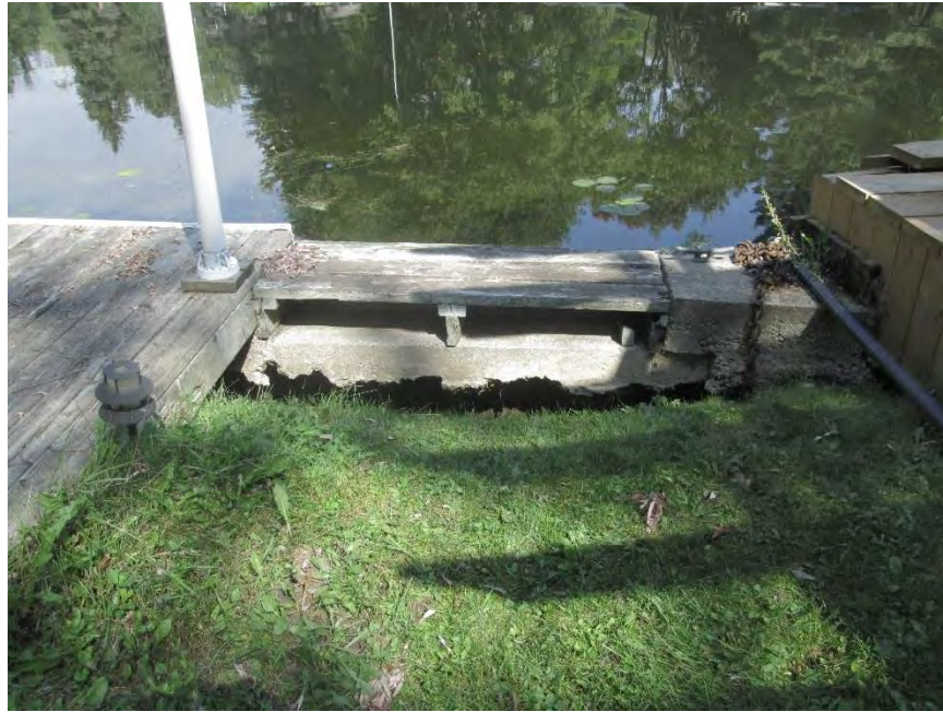
Photograph No. 7 Severe erosion at swale outlet. Swale blocked by constructed boardwalk.
