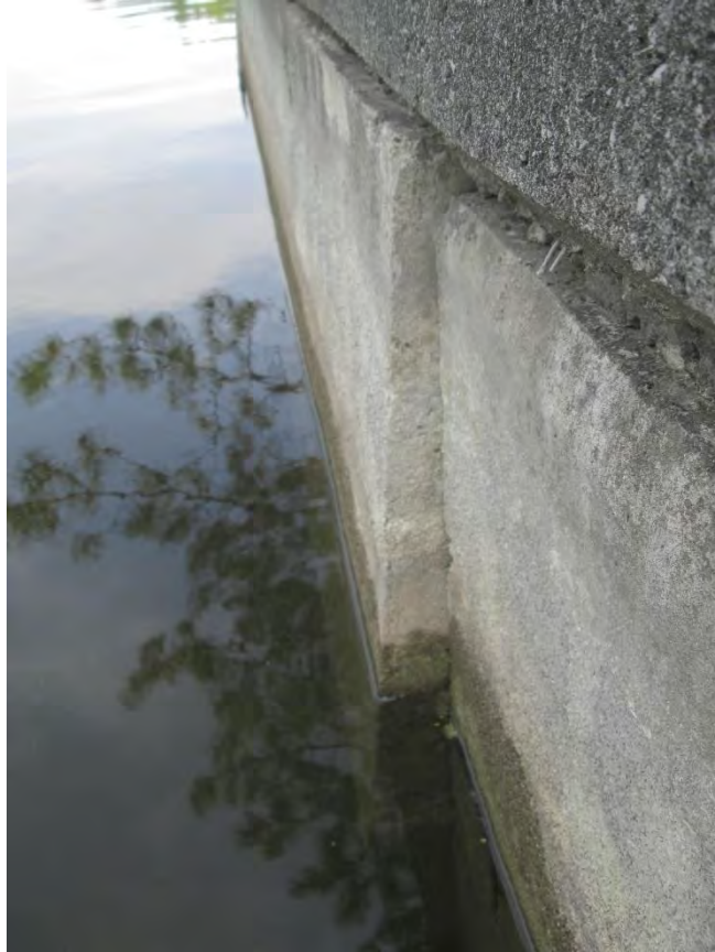
Photograph No. 17 Differential lateral movement of concrete fascia panels.
