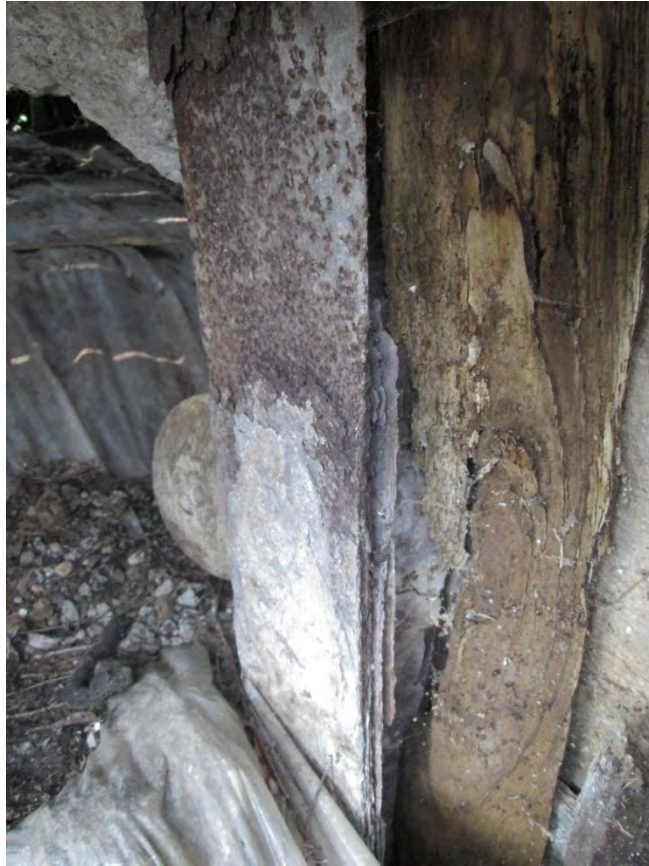
Photograph No. 19 Severe corrosion (flaking) of pile flange.
