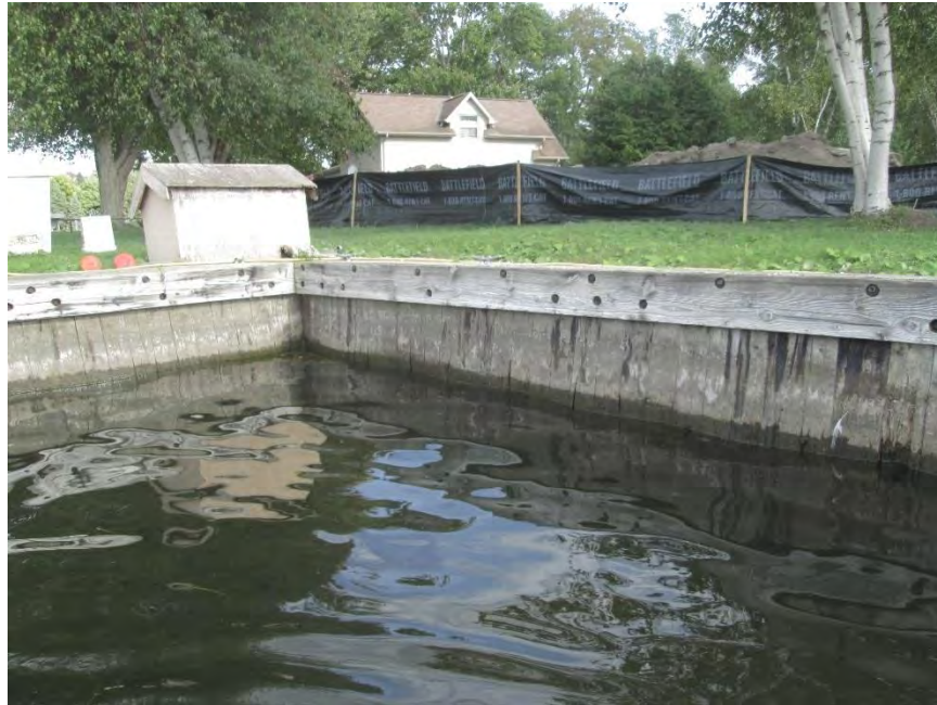
Photograph No. 1 Typical wood plank shorewall.
