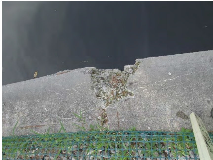
Photograph No. 18 Spalling of concrete cap with exposed rebar.
