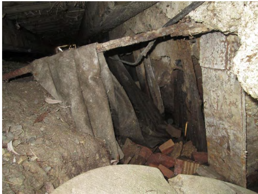
Photograph No. 20 Severe corrosion (flaking) of pile flange and tieback.
