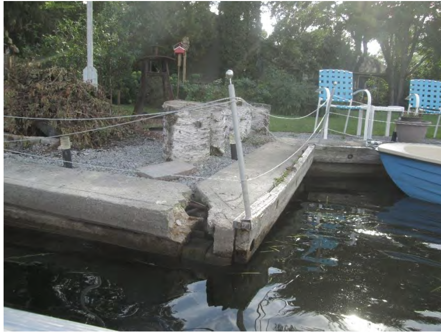
Photograph No. 13 Damaged top cap, exposed rebar and pile – settlement of wall.
