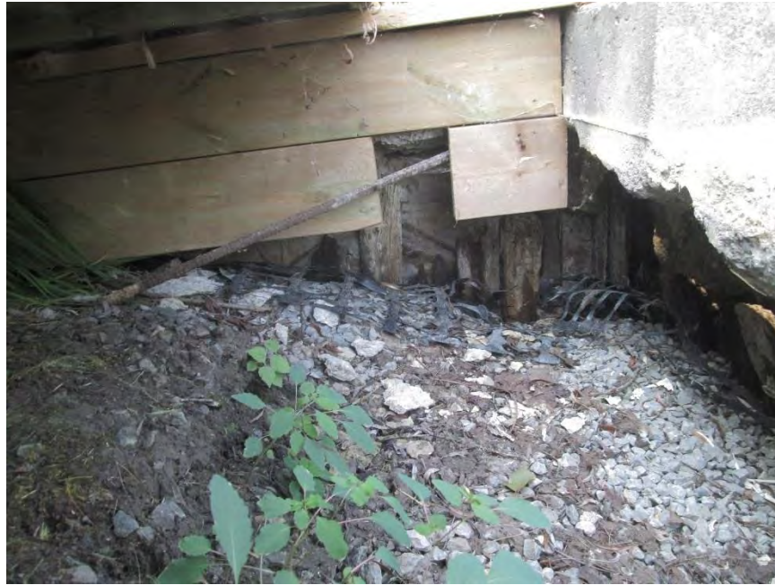
Photograph No. 11 Severe erosion behind wall – exposed piles and tiebacks.
