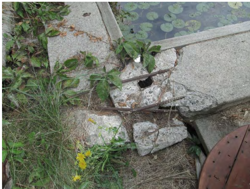
Photograph No. 14 Damaged top cap, exposed rebar and pile.
