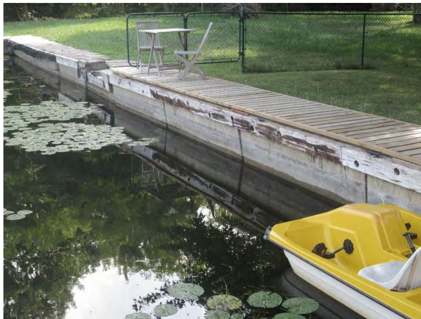
Photograph No. 16 Slight lean in top of wall towards canal.
